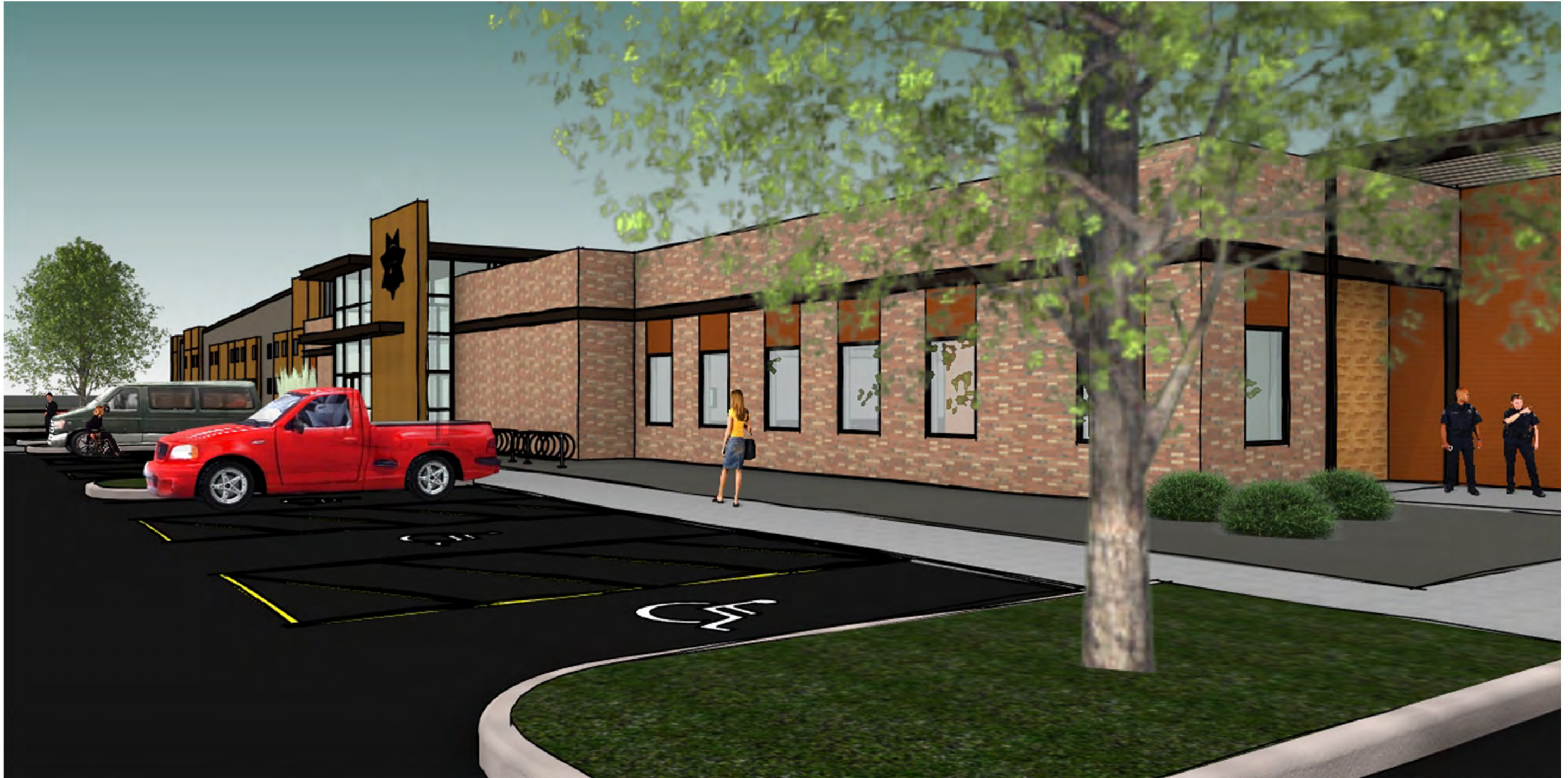
Lewis and Clark County Public Safety Facility - Front Perspective
